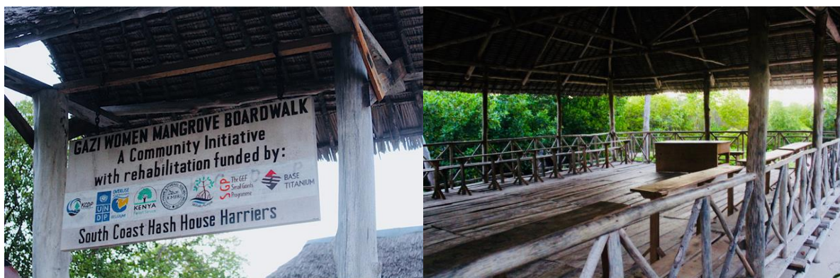
Photo 2: Gazi women ecotourism boardwalk infrastructure (Right: Eco-conference hall)
