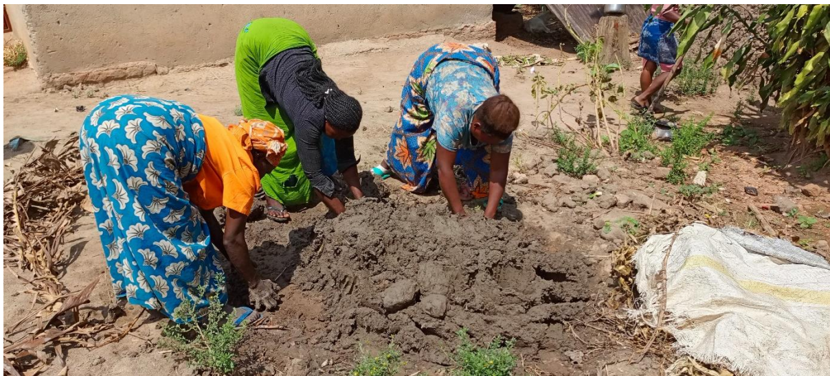
Photo 4: Women preparing the soil for stove construction in Gogonya © by Jjemba (June, 2024)
