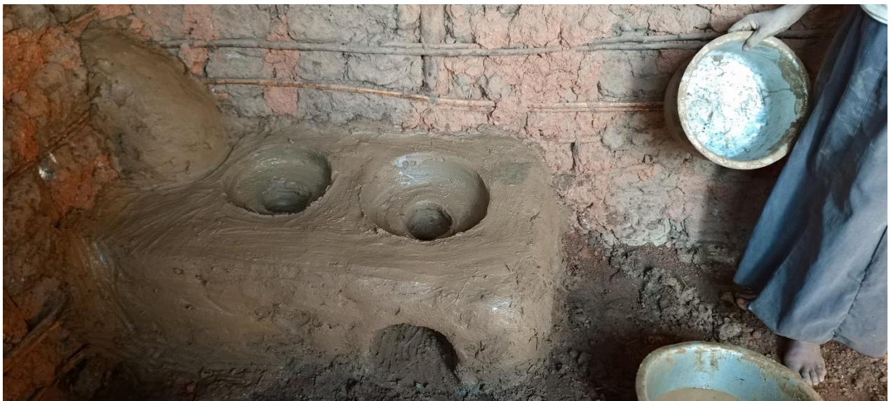
Photo 6: A constructed Lorena stove in a local kitchen in Gogonya © by Jjemba (June, 2024)
