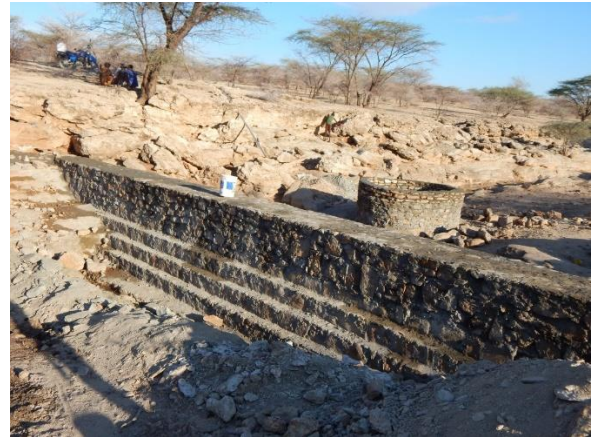
Finished sand dam wall
