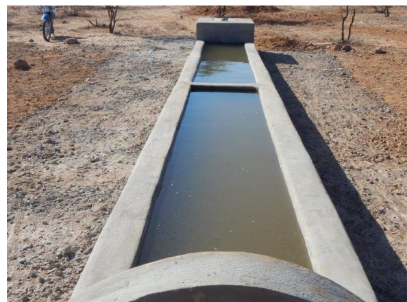
Completed wildlife trough 450m from the river
