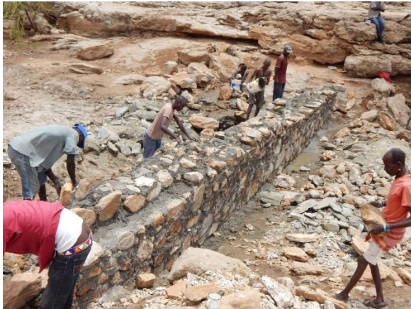
Building the sand dam wall
