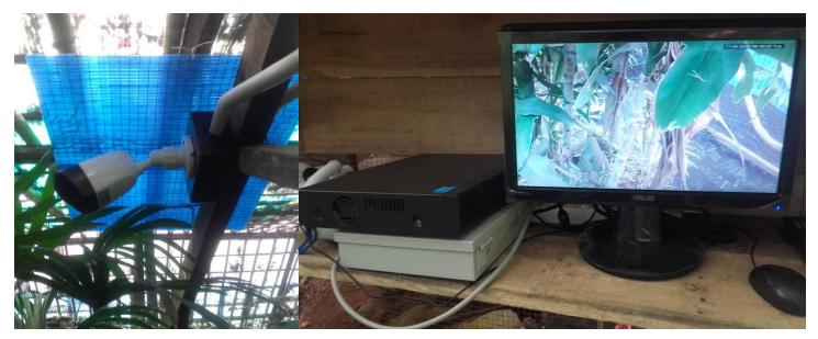
Picture 4. CCTV system installed in one of our buildings: High-resolution camera with cables protected into safe box and PVC pipes (left). Screen and electrical installation protected against lightening (right)
