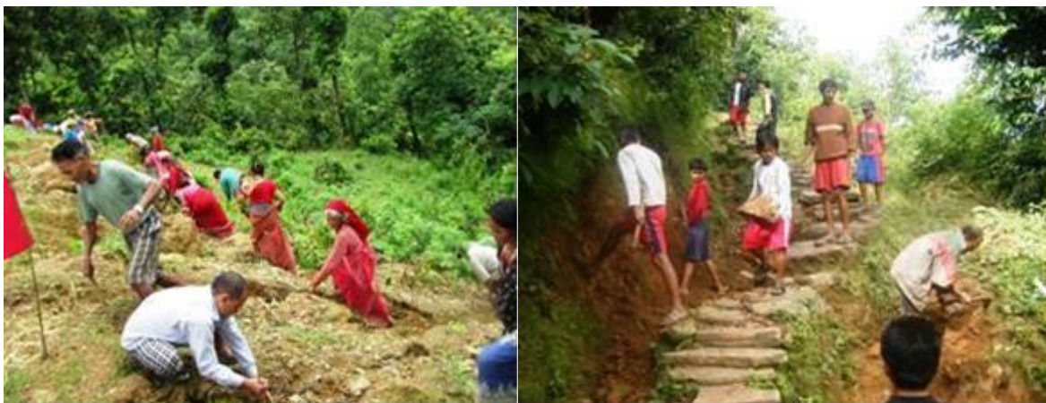
Left: Farmers, Boaters and Fishermen in plantation event in Pachabhaiya, Rupa watershed. Right: Watershed area rehabilitation work in Begnas watershed with community involvement.
