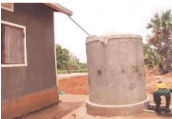
Left: Rain water harvesting tank (concrete) at Nakasongola SSS. A similar one was erected at Kirojo College
