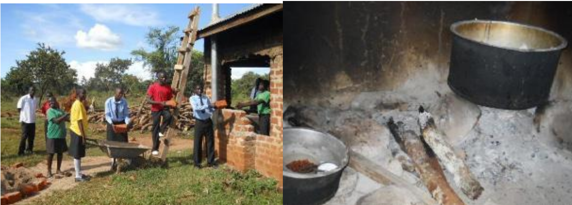
Left: Kirojo College School Students participate in the construction of energy-saving stoves; Right: Status of energy-wasting stove before construction of energy-saving stoves
