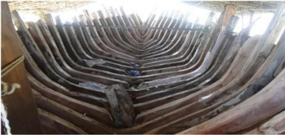
Interior of the Ozi Beach Management Unit boat as it was being constructed in April 2011
