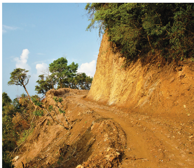
79. Road construction cutting through a section vulnerable to erosion and landslides.
