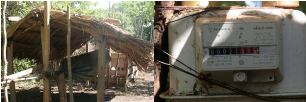
Left: Biogas storage tank. Right: Gas meter for evaluating biogas production.
