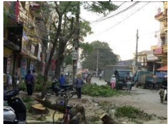
The clearance of attached trees for wider road
