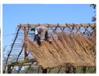
Constructing and thatching the main shade banda at the new RCP field camp
