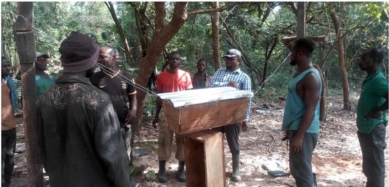
Plate 4. Hands-on training by Dr. Ishmael Hashmiu on beehive fence installation. Credit: Ishmael Hashmiu
