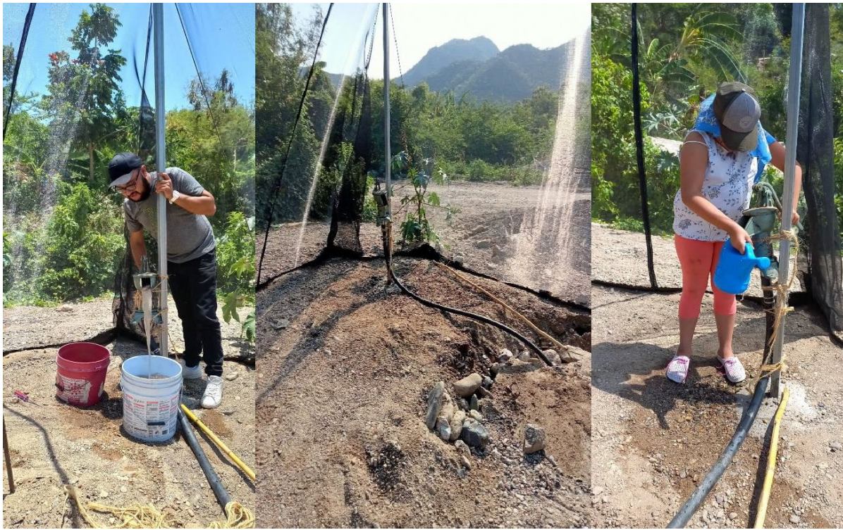
Installation of the deep well water extraction manual pump
