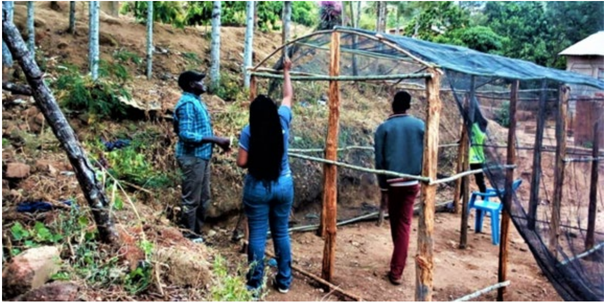
Figure 4: Installation of 75% black shade-net around the external wooden frame
