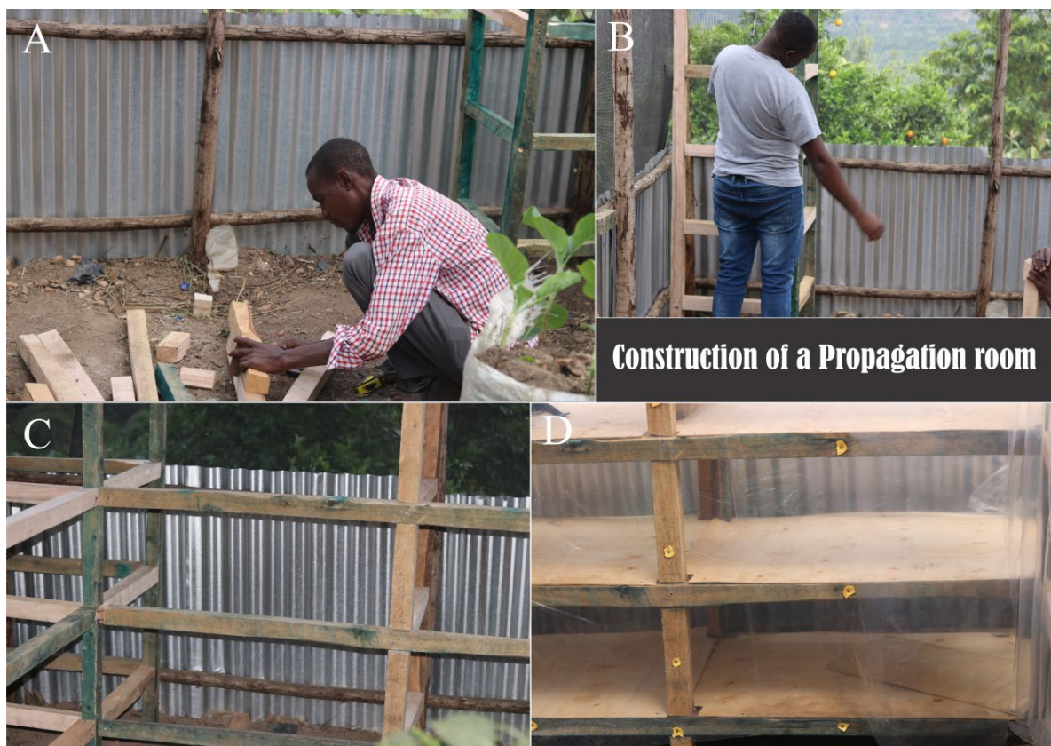
Fig. 1: Establishment of a propagation center. A - Carpenter cutting wood pieces into required sizes, B - the project leader confirming the height measurements for the propagation shelves, C - Propagation shelves fitted into the propagation room, and
