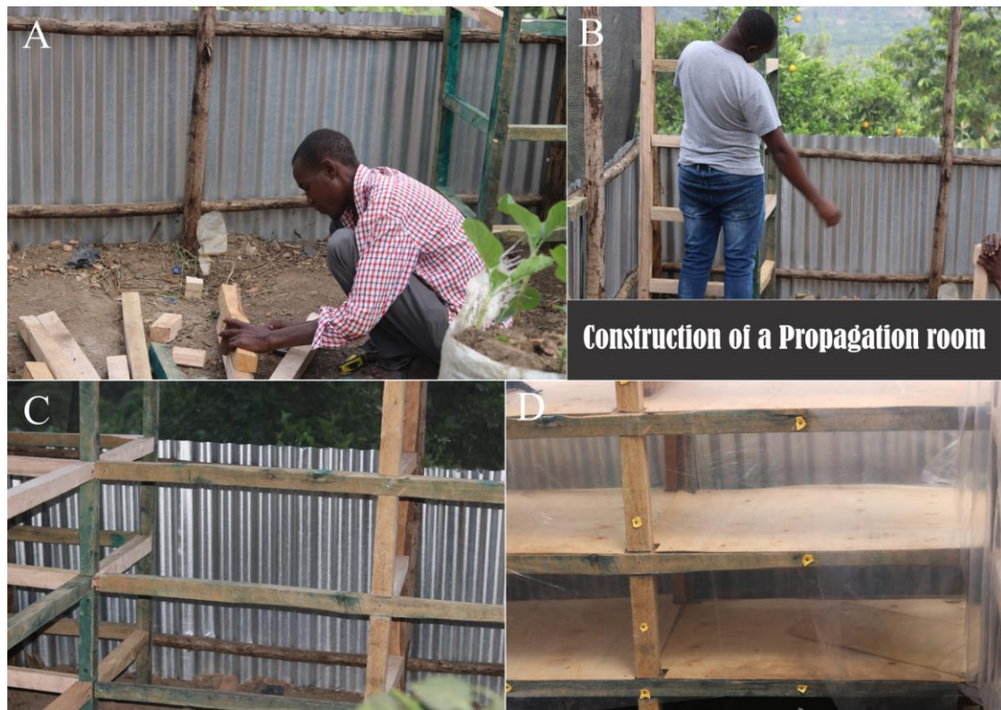
Fig. 5: Establishment of a propagation center. A - Carpenter cutting wood pieces into required sizes, B - the project leader confirming the height measurements for the propagation shelves, C - Propagation shelves fitted into the propagation room, and D - Propagation shelves fitted with ply wood partitions and clear polythene for light regulation.
