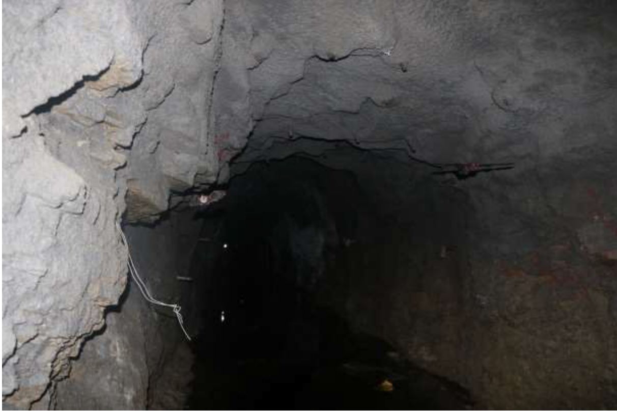
Figure 4: A hydropower testing tunnel serving as a roost for Hipposideros gentilis and H. armiger , Dolakha
