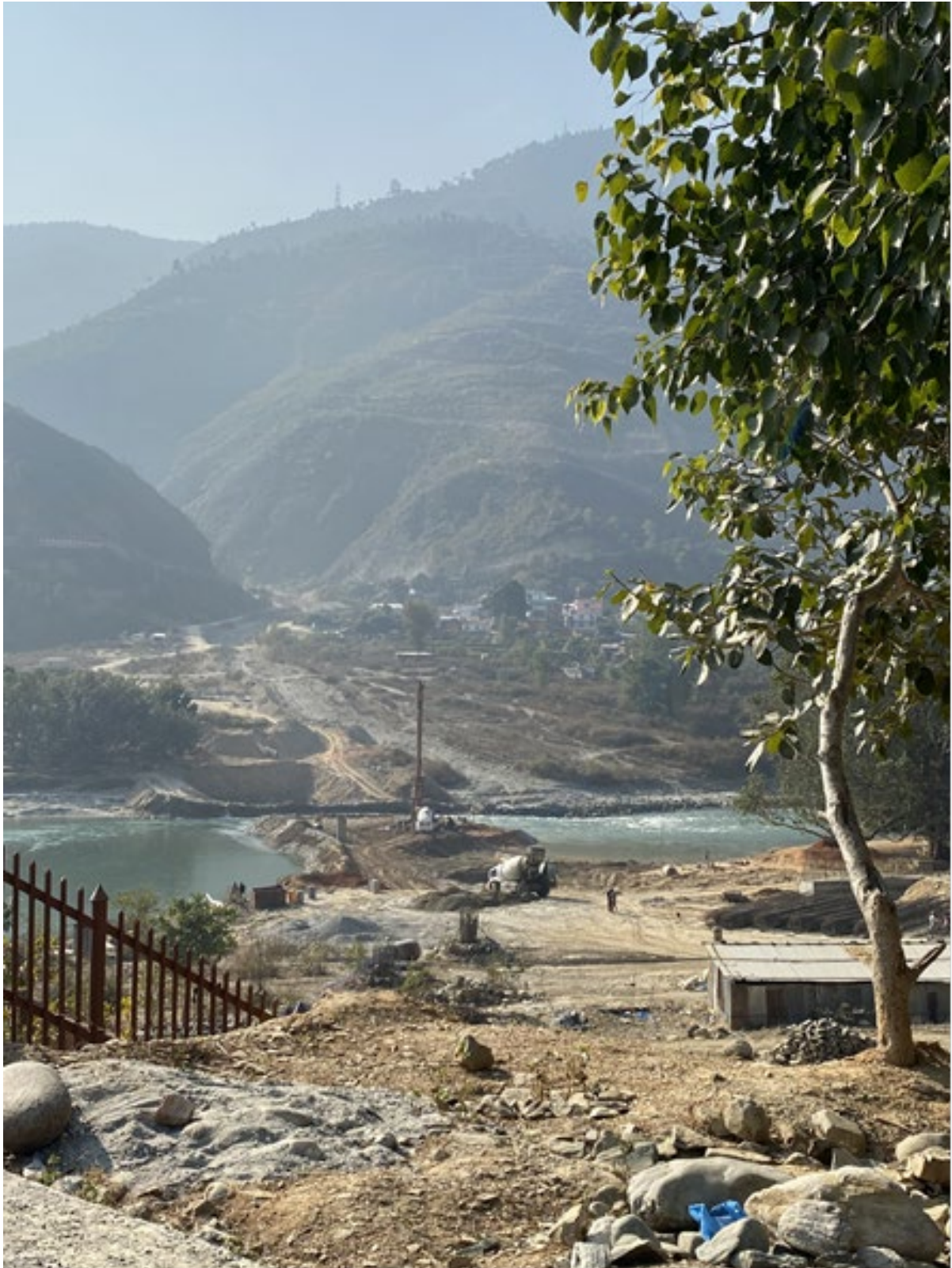
Figure 20: Bridge construction on the Tamakoshi River in Manthali, Ramechhap district.
