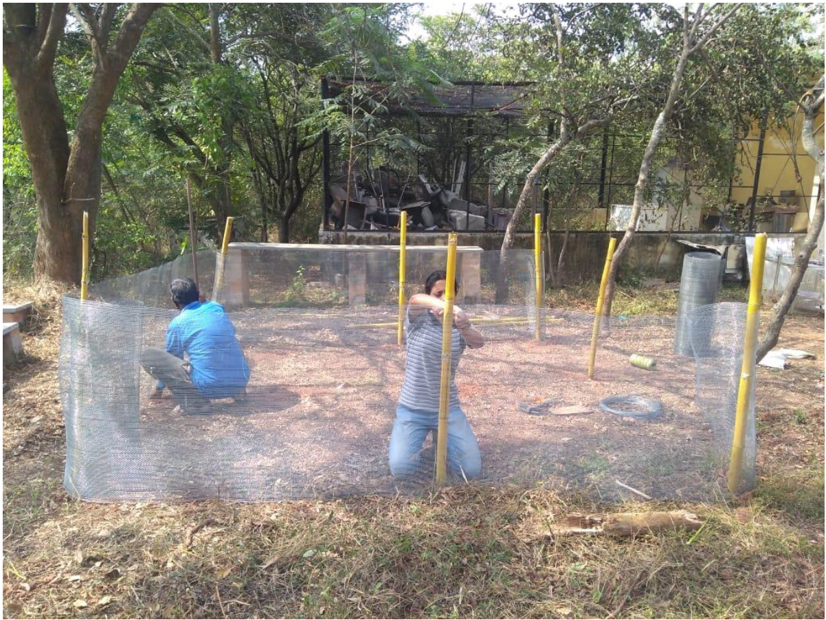
Initial enclosure construction
