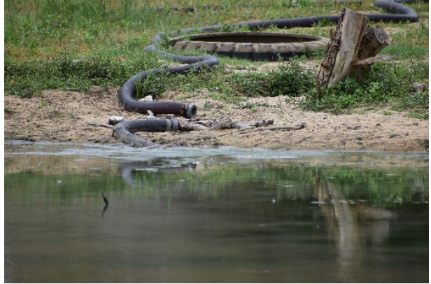
Water abstraction at Lango la Simba wetland for road construction
