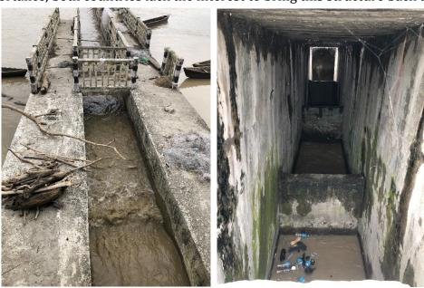
Picture 15: Fish ladder at Koshi barrage; non-functioning at the moment
