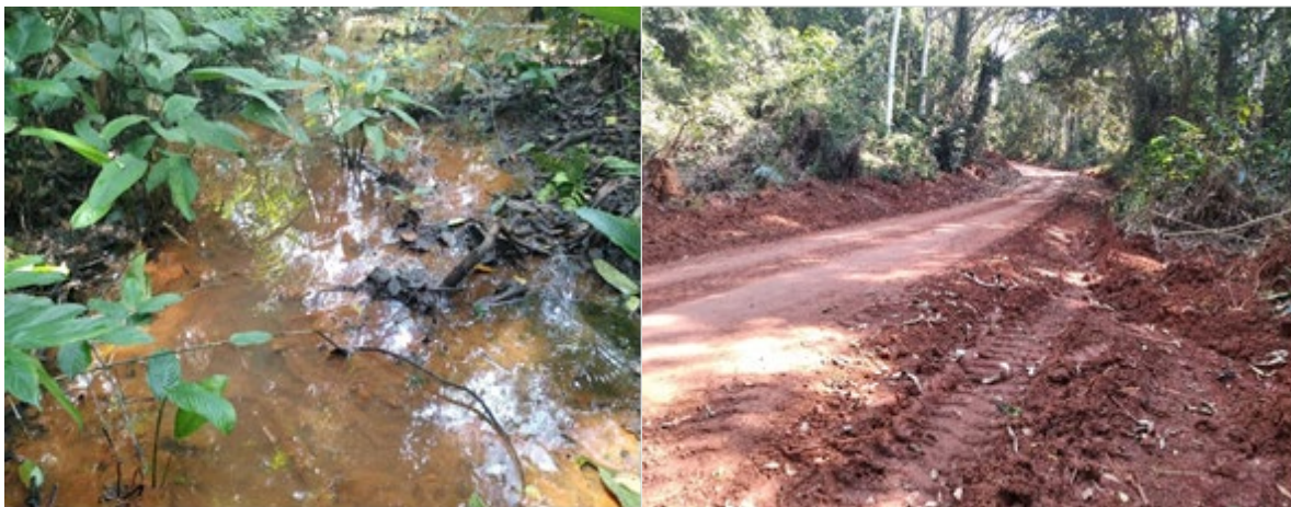
Left: Water pollution in DDNP. Right: Road infrastructure in DDNP.
