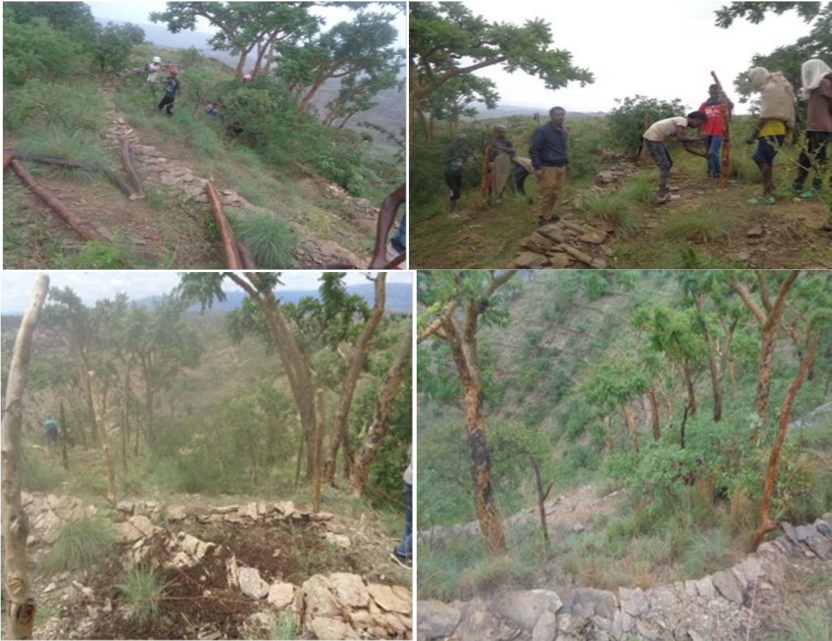
Figure 4. Established soil and water conservation structures inside of the degraded habitats of B. papyrifera tree species.
