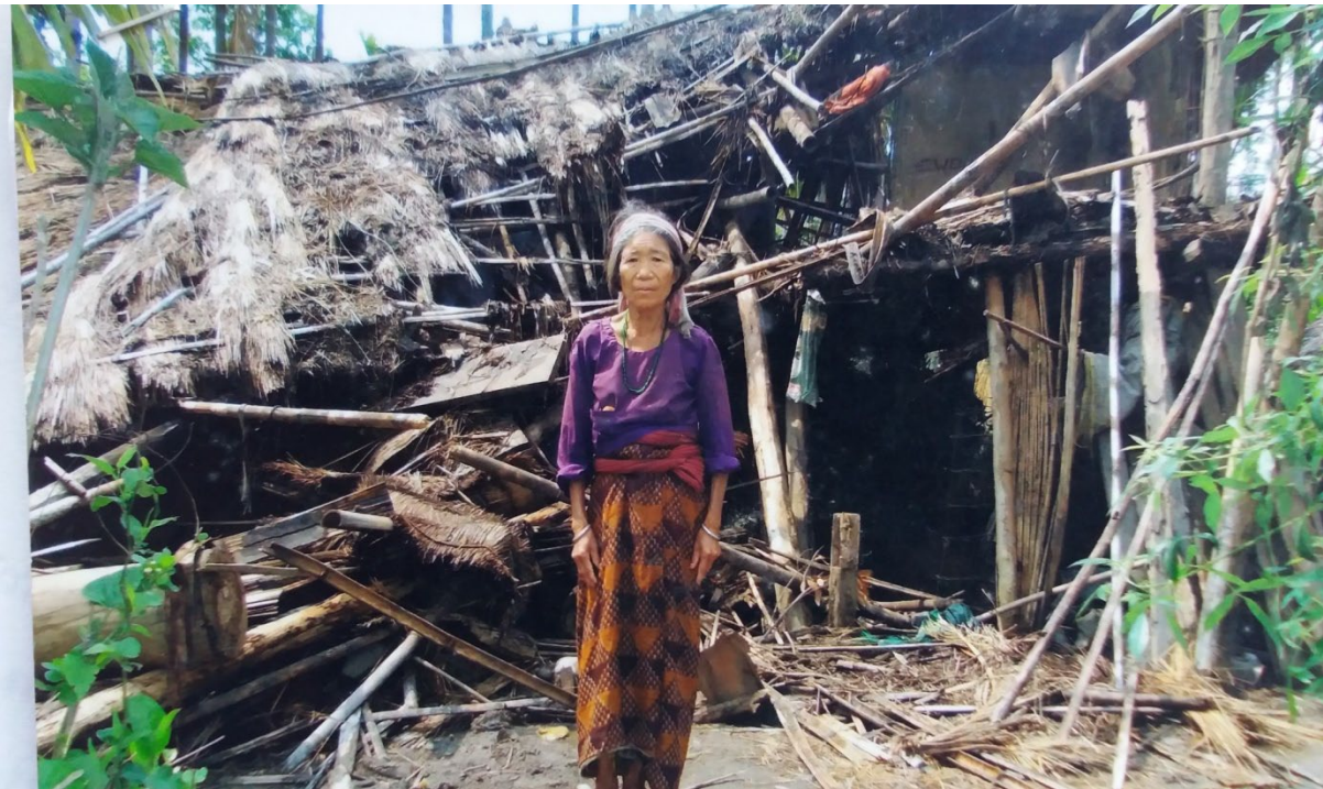
Fig House damage by elephants
