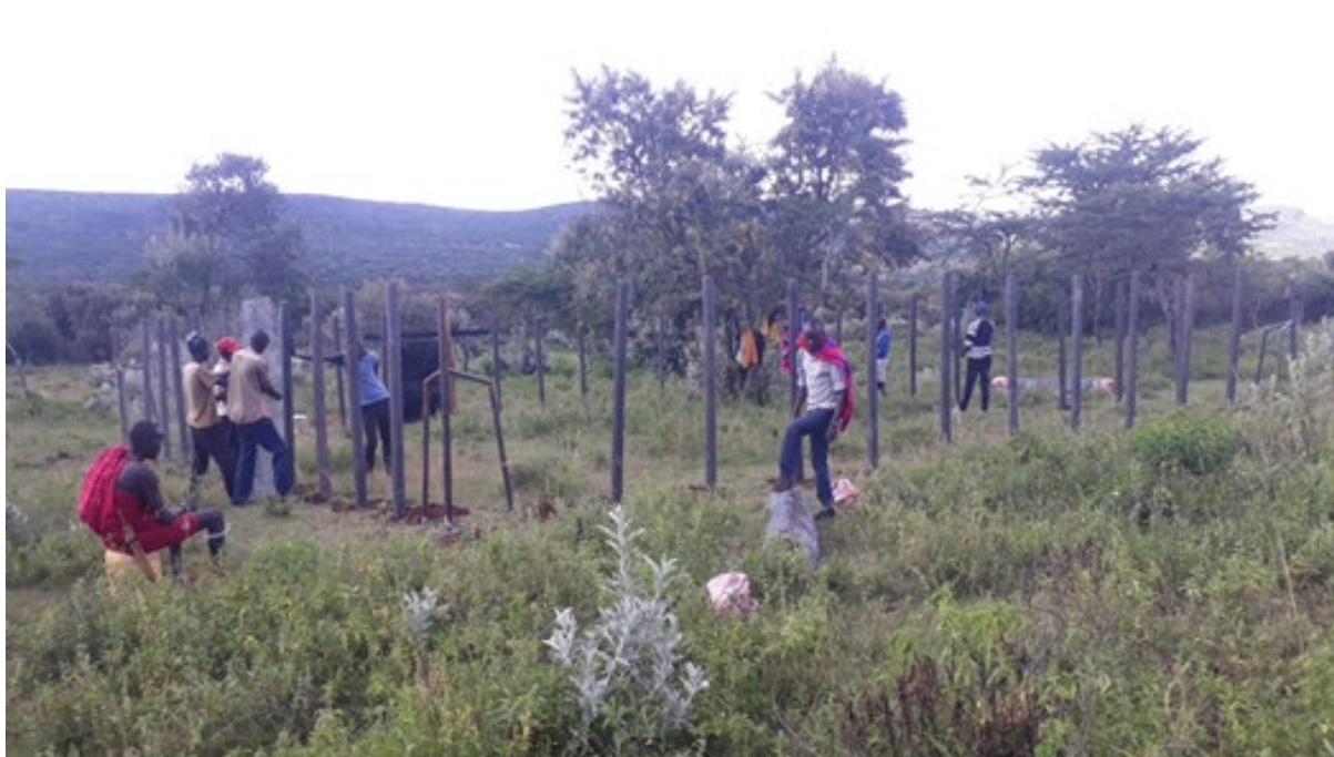
Figure 1: Construction of predator proof Kraal/Boma in Siana conservancy
