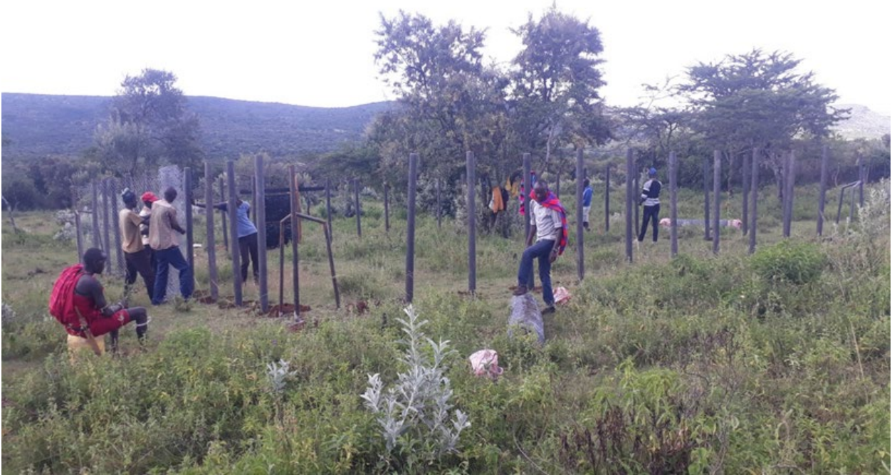
Plate 1: Construction of predator proof Kraal/Boma in Siana conservancy
