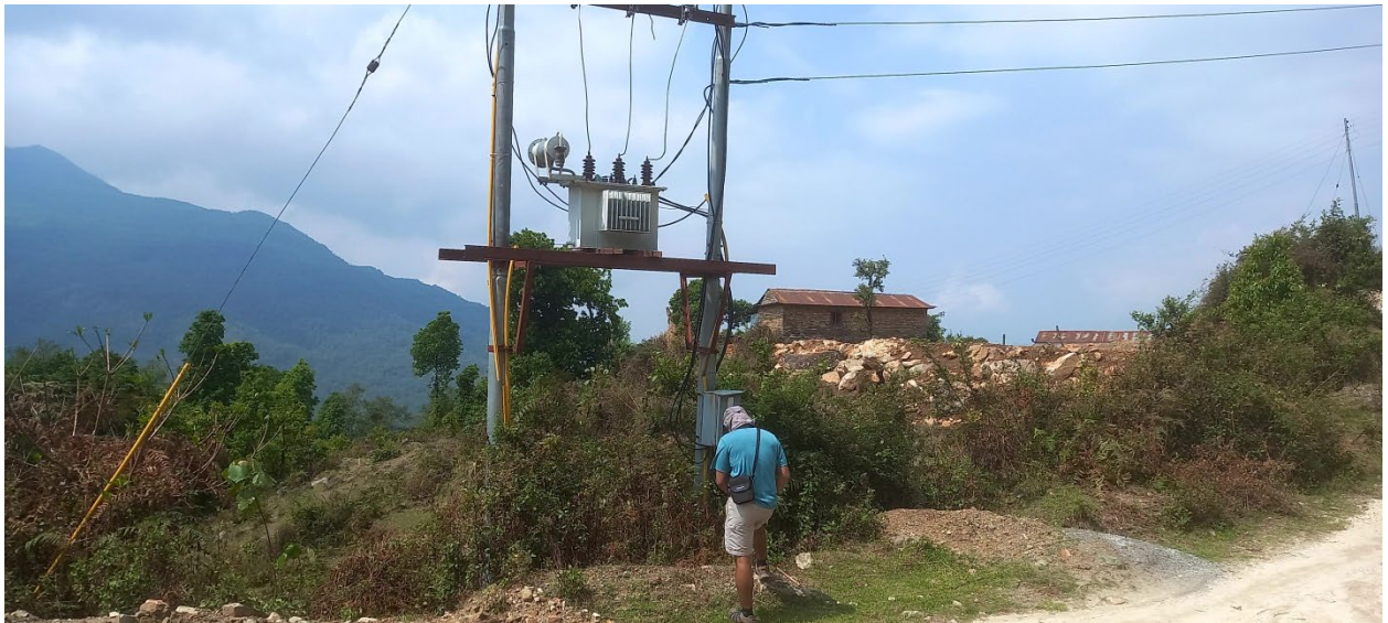
Photo 9: Researcher recording the design of the power lines (Horizontal H-frame with a switch and transformer)
