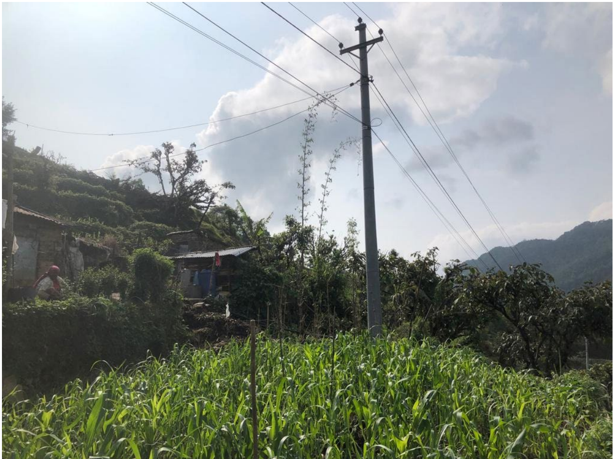
Photo 7: Triangular configuration power lines with a simple pin-type insulator in Chitre, Parbat
