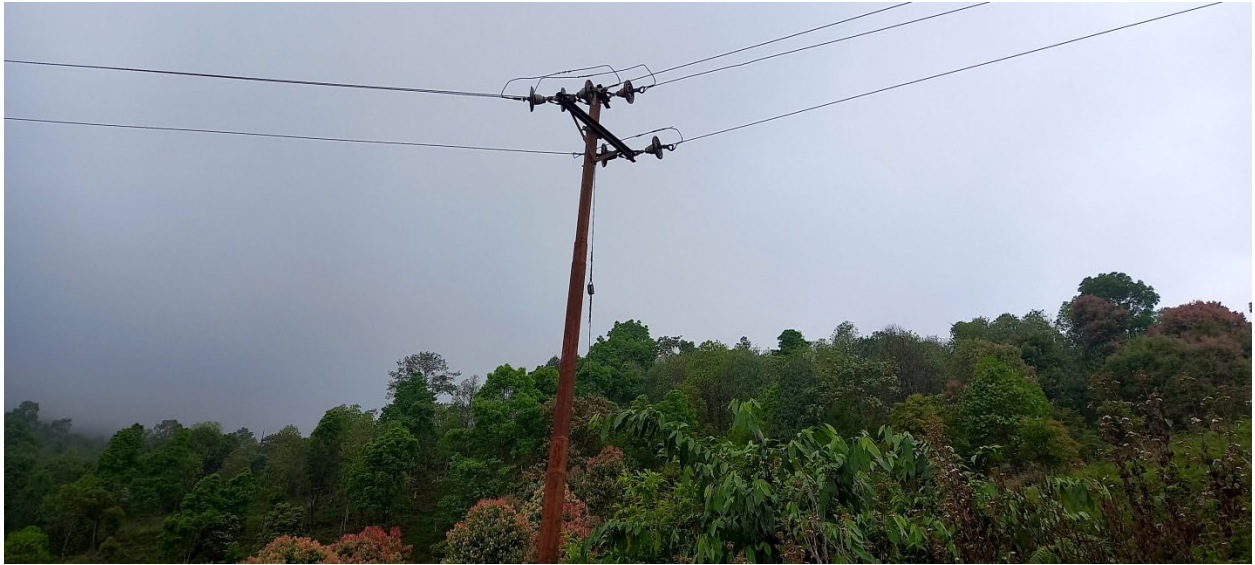
Photo 8: Triangular configuration power lines with a jumper on it
