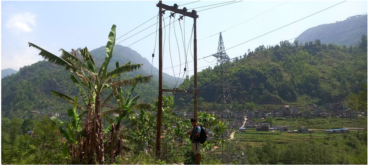
Photo 6: Simple H-frame with a strain insulator with a Double circular angular strut design high transmission line behind at Nayapul
