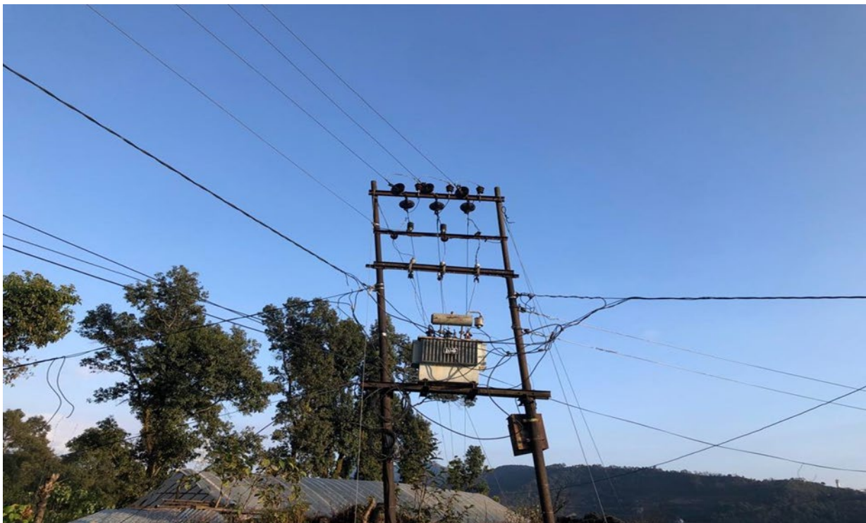
Photo: Horizontal configuration with a "Simple H-frame" with a ceramic insulator arranged in "strain insulator" type with an external transformer
