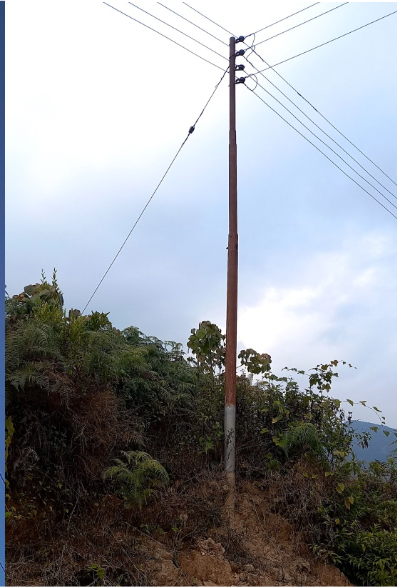
Photo: Triangular configuration with "Simple I" cross-shaped having a cross arm made of metal (left) and vertical configuration with an absence of cross-arm materials (right)
