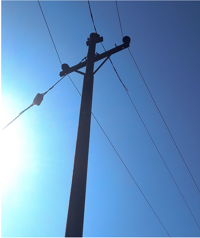
Photo: Triangular configuration with "Simple I" cross-shaped having a cross arm made of metal (left) and vertical configuration with an absence of cross-arm materials (right)
