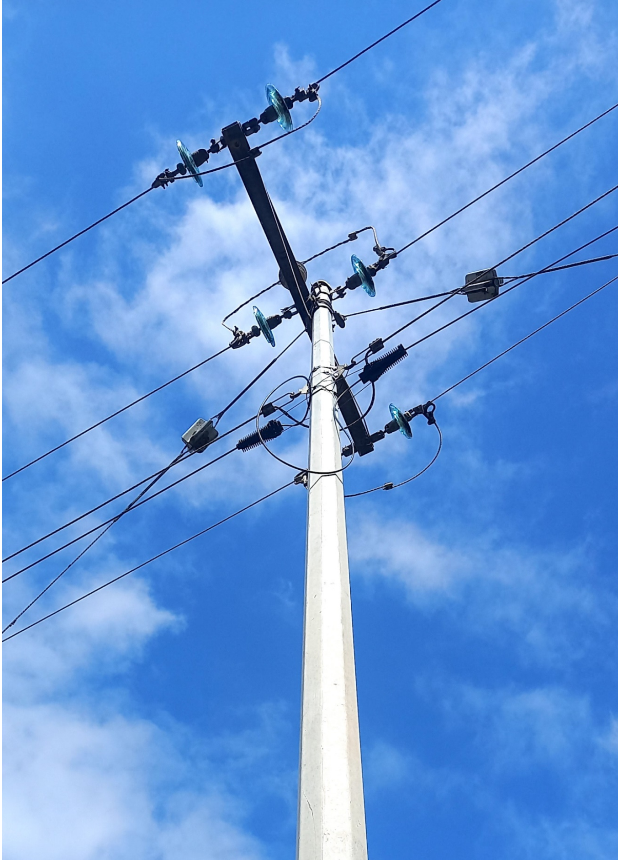
Photo:" Simple I" type of Horizontal configuration with a glass insulator "strain insulator" arrangement having 3 jumpers about the insulators
