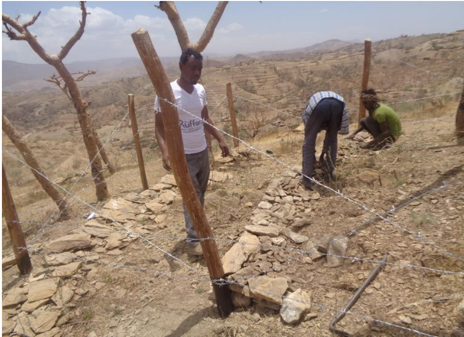
Figure 4. Introducing soil and water conservation structure (traces using stones) inside of the established area enclosure with stakeholders for assisting natural regeneration of Boswellia papyrifera
