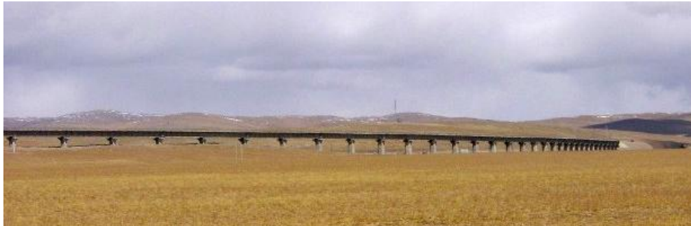
Fig 9. Budongquan Wildlife Passage
