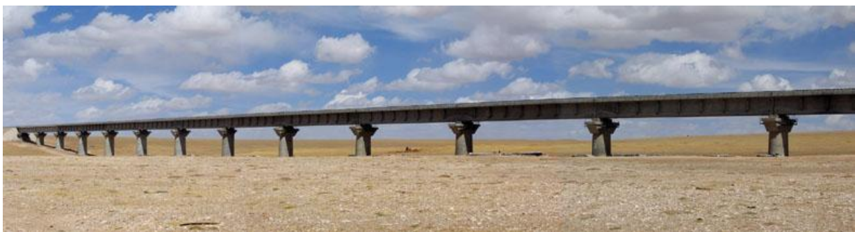
Fig 7. Wudaoliang Railroad Bridge
