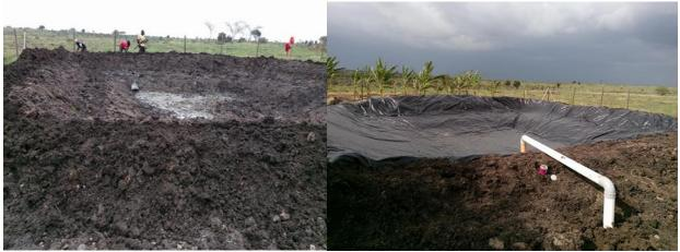
Left: Compaction of the soil to ensure stability. Right: Installation of water inlet into the pond.
