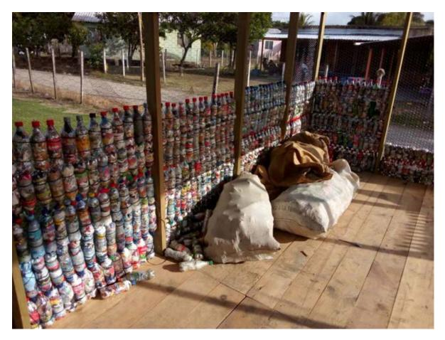
Once all the walls are filled with ecobricks, they will be covered with a layer of cement that will protect the chicken wire against the salt of the ocean
