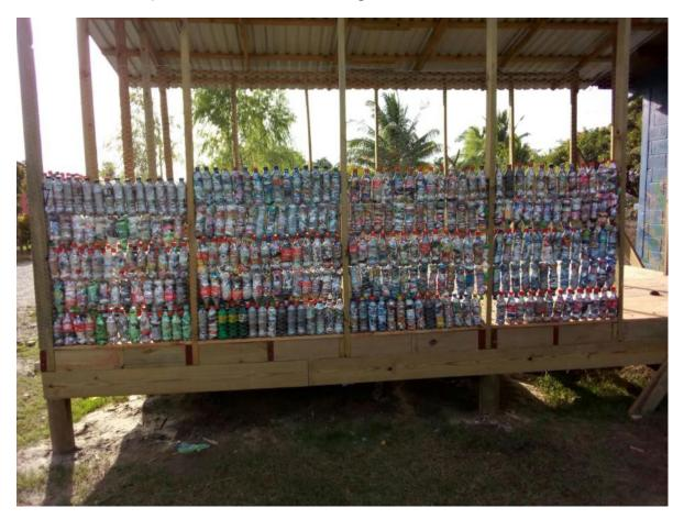
Spaces between walls will be also filled with more plastic trash before they cover the walls with cement.
