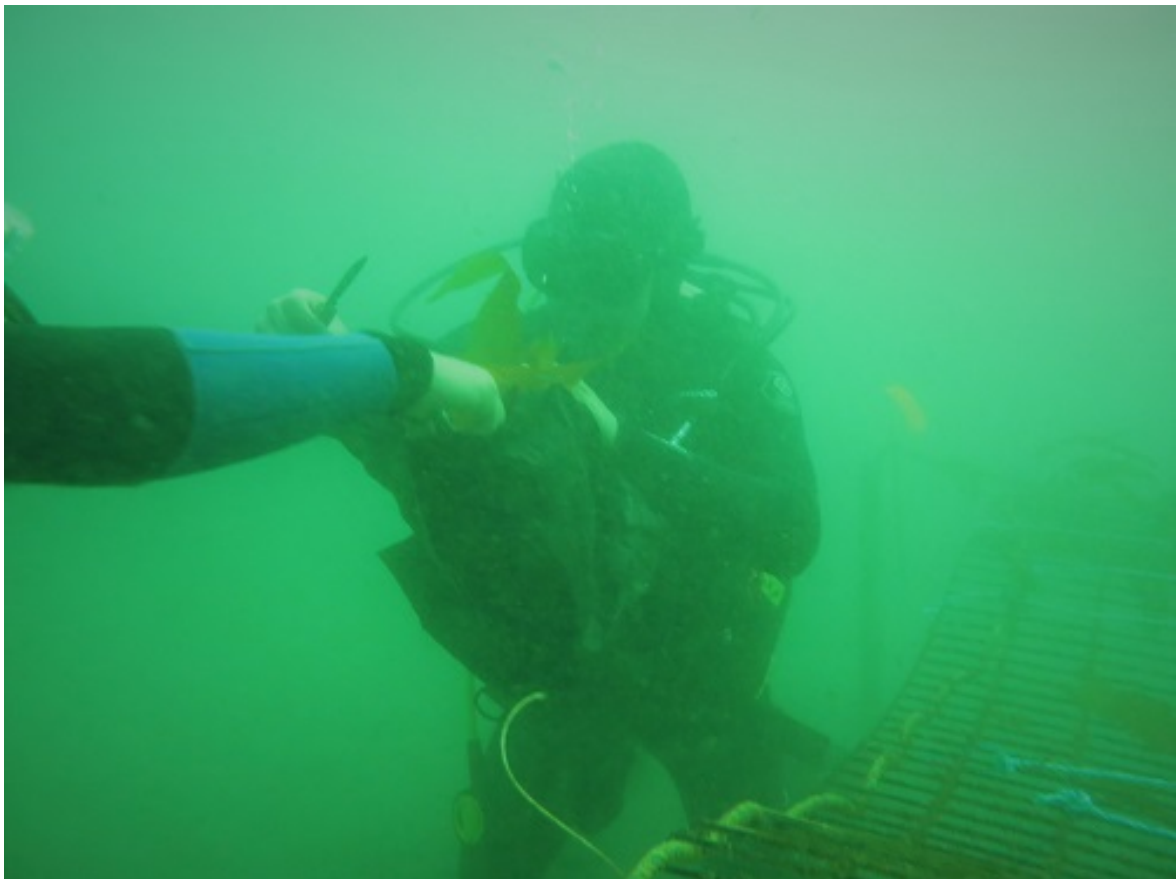
Bringing young algae to be installed on the structures.
