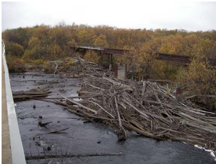
Fig. 9. Collapsed bridge across the Dagi River. A number of trees washed away by floods have accumulated between the bridges.
