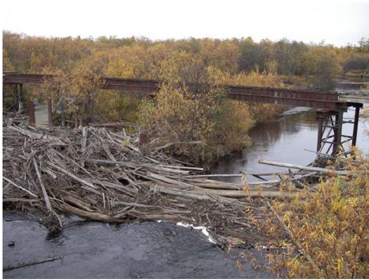
Fig. 8. Bridge across the Dagi River. This is the abandoned Nogliki-Okha railway line. Large accumulation of the logs as a result of floods is clearly visible under the bridge.
