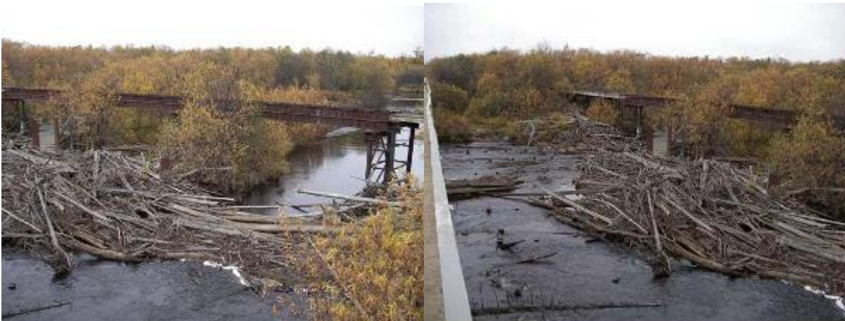
Fig. 8. Bridge across the Dagi River. This is the abandoned Nogliki-Okha railway line. Large accumulation of the logs as a result of floods is clearly visible under the bridge. Fig. 9. Collapsed bridge across the Dagi River. A number of trees washed away by floods have accumulated between the bridges.
