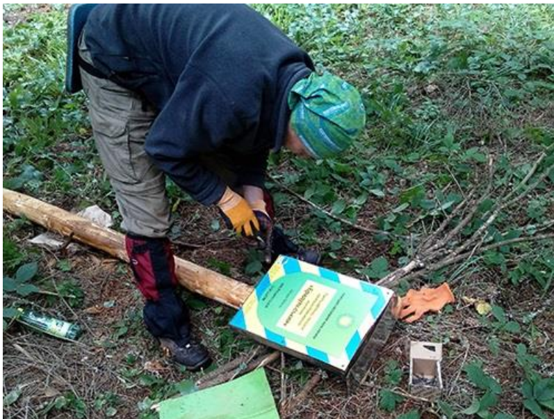
Installing boundary sign
