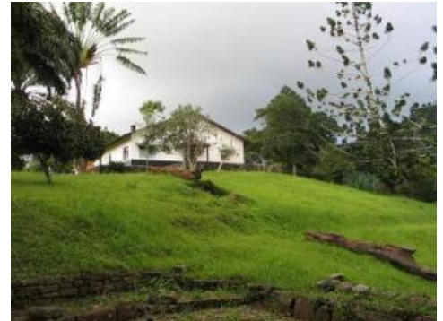
Figure 38. Estate manager's house.
