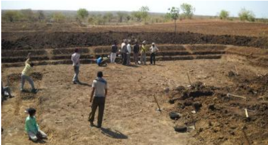
Figure 4: Eco-restoration work going on at Kajaleshwar Village.
