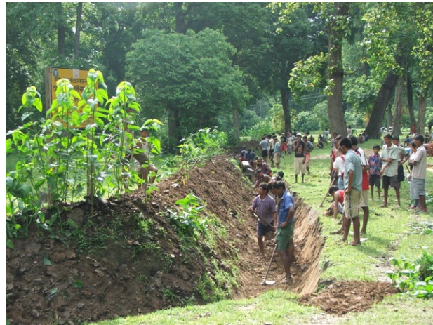
Figure 8. Collective action from communities for trench construction.
