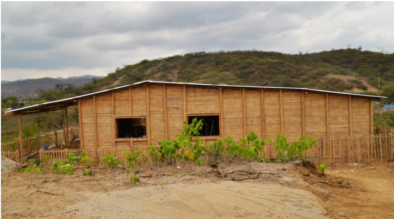
Interpretation Center built in Rica Playa town, in the buffer zone of the Noroeste Biosphere Reserve
