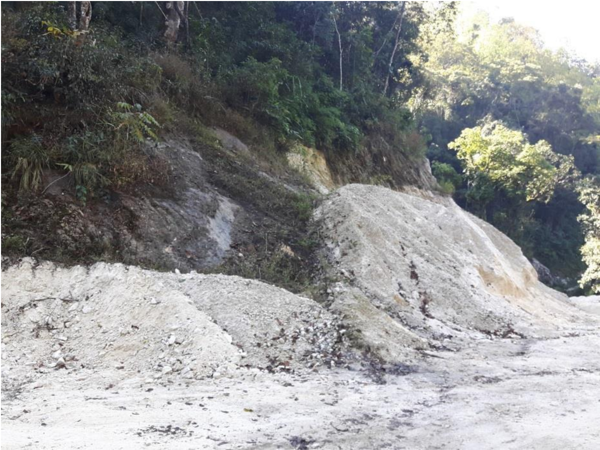
Figure 3: The construction of farm roads along Paphiopedilum fairrieianum habitat.
