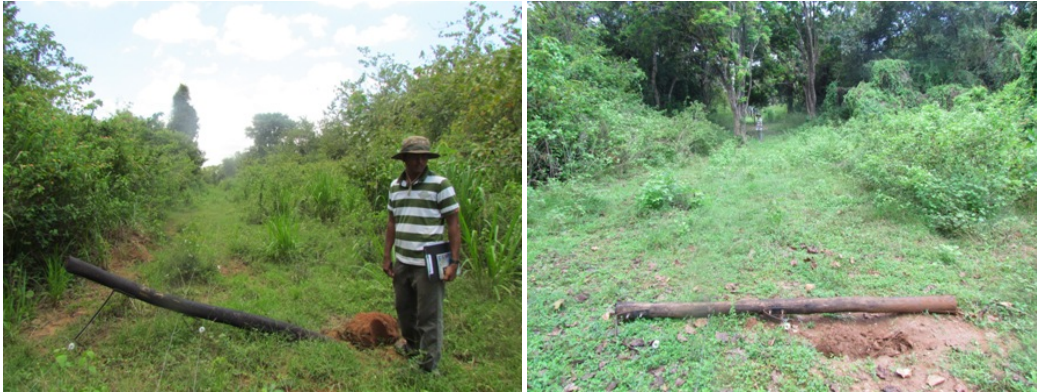
Plate 5: Fallen posts of the park electric fence.
