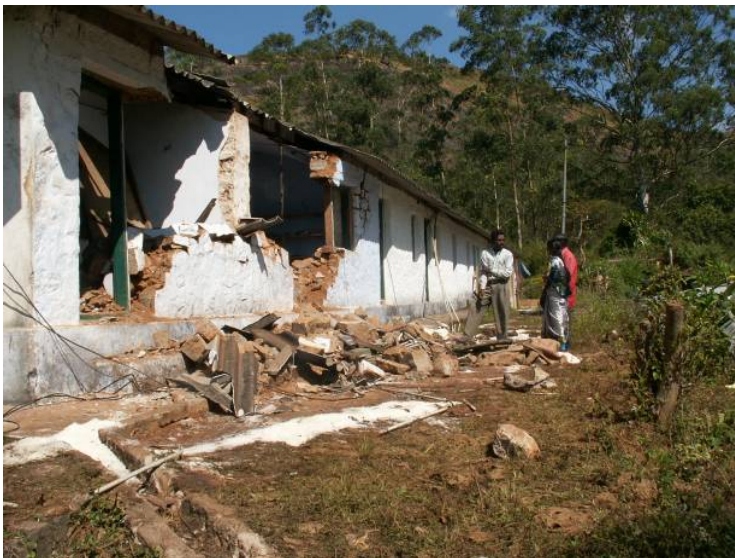
Presence of ration shop in human habitations may cause damages to residential places (In picture: Ration shop along with houses damaged by Monica herd in one of the Tata coffee estates of the Valparai plateau).
