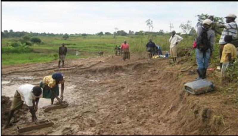
Plate 3 Brick-laying activities being carried out along trail 3.
