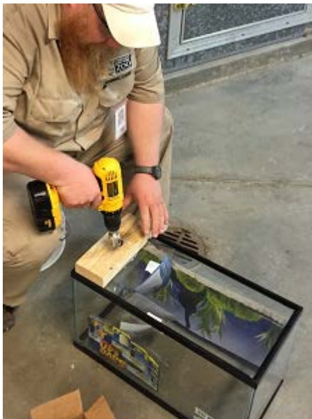
Glass aquarium tanks are modified for assembly onto the amphibian husbandry rack system. ©Nathan O'Brate
