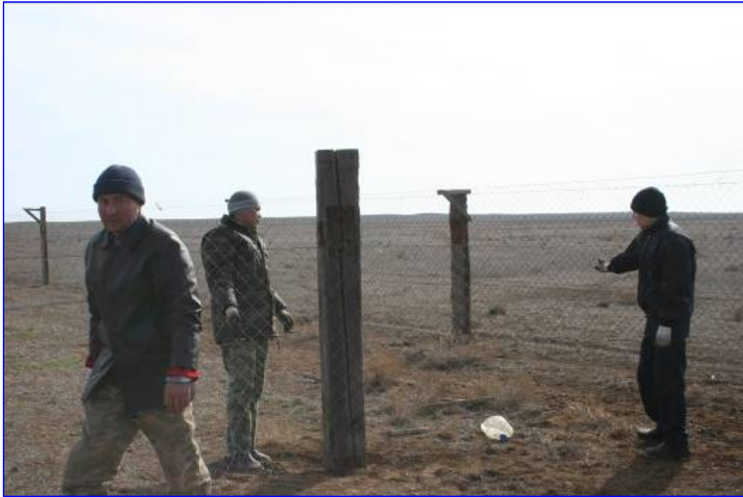
Repairing old enclosure (Photo Yuriy Arylov)
