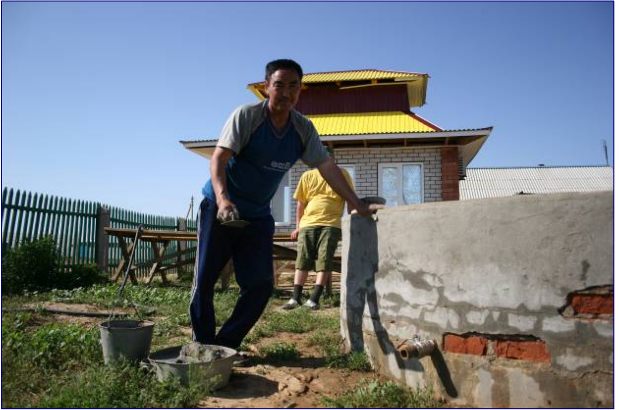
Rebuilding of water storage (Photo Yuriy Arylov)
