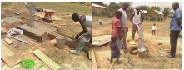
Left: A mason working on the newly constructed borehole. Right: Newly constructed borehole operated by a hand-held water pump. © Dinfa Barshep.
