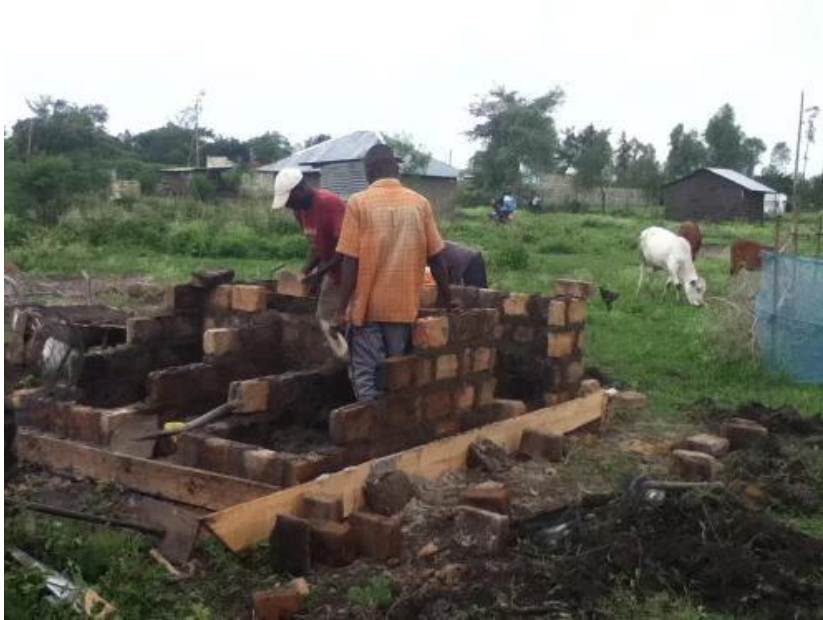
Photo 5: A double vault ecosan toilet under construction.
