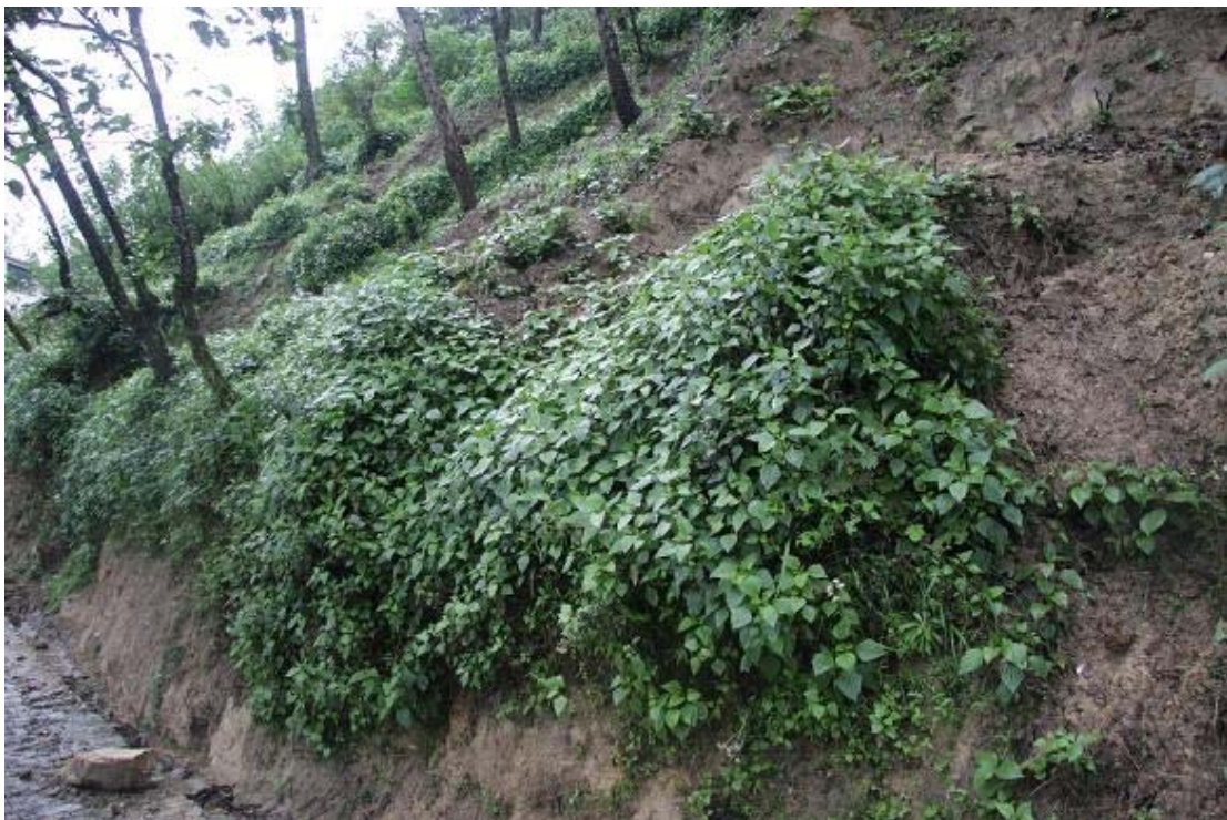
Fig.8.4. Croftonweed and the loose soil
