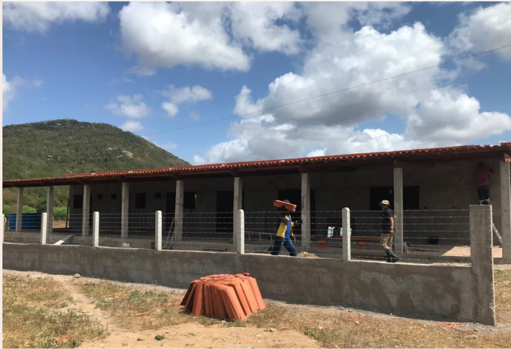
New Building of the SOS Caatinga Institute under construction.
